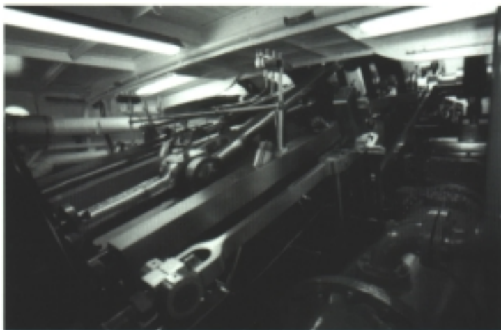
View, looking aft, of the engine's crossheads, rods and valve gear. The two cylinders are just out of sight to the left. The condenser is to the right. Photo: Kurt Bieri, Rothenburg
